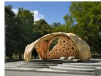
Fig: 8 The project explores the architectural transfer of biological principles of the sea urchin's plate skeleton morphology by means of novel computer-based design and simulation methods, along with CNC methods for its building implementation
