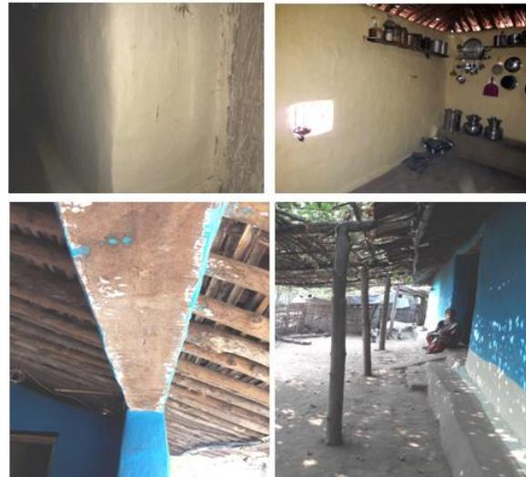
Figure 8 Mezzanine floor, timber truss with country tiles and staircase made out of mud
