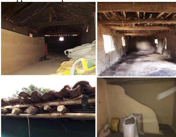
Figure 7 Thick wall, finished floor, wooden lintel and raised plinth of the house
