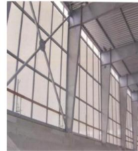
Figure 2 Aerogel glass wall (Kroto & Veith, 2008)
