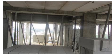
Fig. 2.4 Placing of beams with better supporting system
