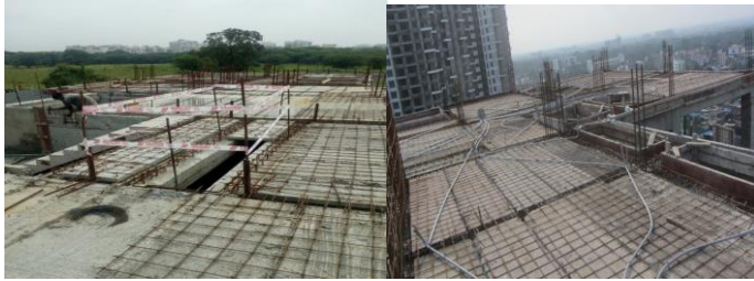
Fig 2.5 Placing of slabs
