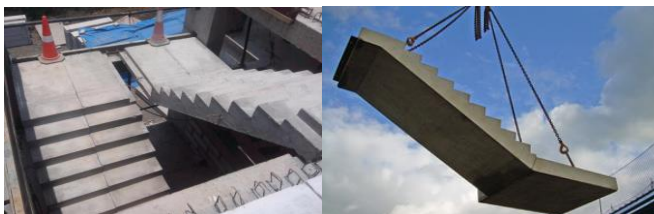
Fig. 2.6 Placing of staircase with hooks to lift and place.
