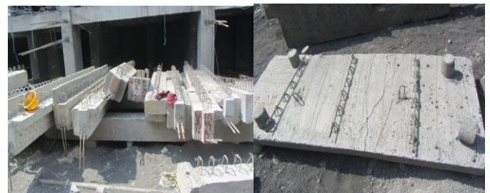
Fig. 2.1.1 Result of Wrong Stacking Work.
