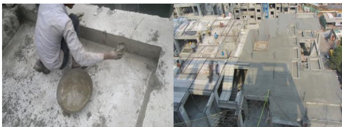
Fig.2.5.2 cement slurry applied in sunken portion to avoid leakages.
