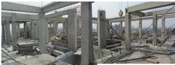
Fig.2.2.2 Supports provided to the column
