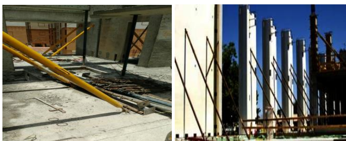
Fig. 2.3 Placing Of Wall and Their Supporting
