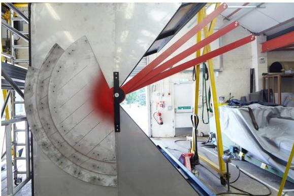
Figure 2.A b: Central steel pivot for opening & closing of Kiosk
