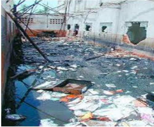
This photo shows the top floor of the building. After consuming the fire the class room partitions and the roof. Here there is no door, window, proper ventilation or escape routes for each class room.
