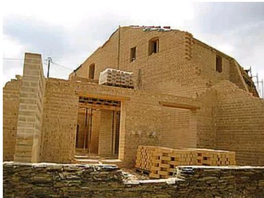
Fig. 2: Structure built using compressed earth blocks (Compressed Earth Blocks-Living Building Material)
