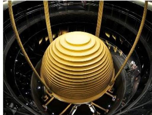
Fig. 3 Tuned mass damper installed in Taipai Tower
